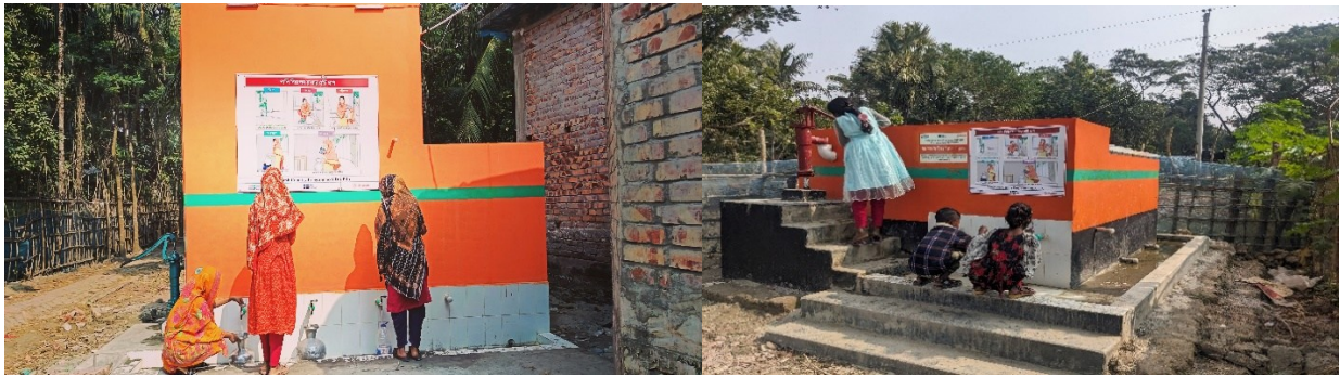
Community people using the pond sand filter to collect safe water
