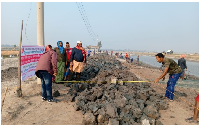
SSM work at Paikgachha, Khulna
