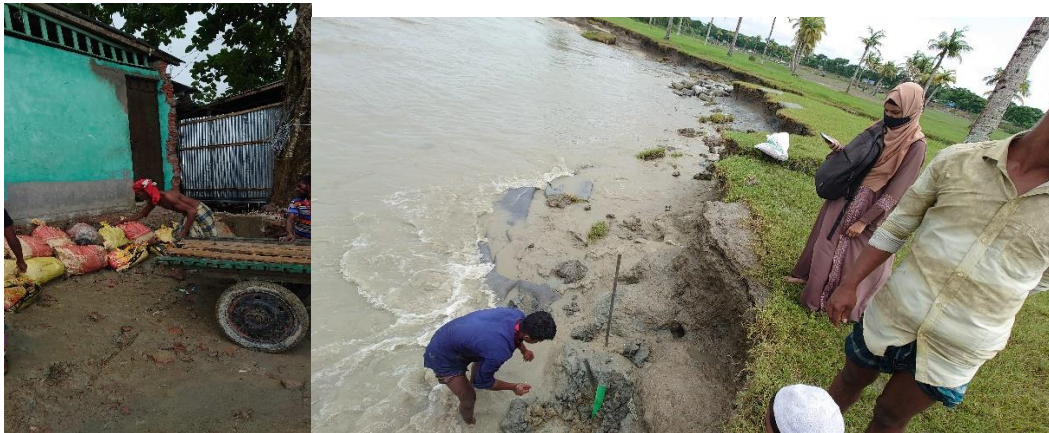
Erosion in study area
