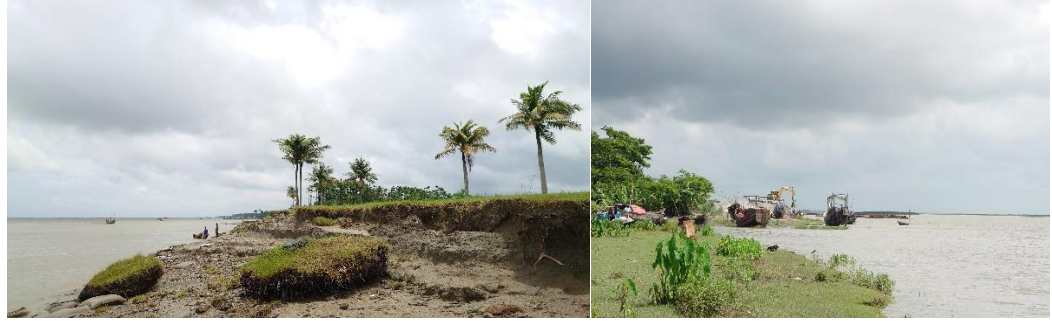
River Erosion in Meghna River (left) in Tetulia River (right)
